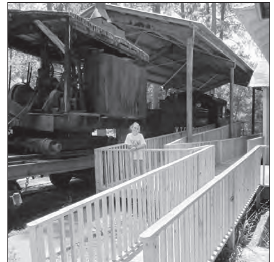
The new ADA ramp makes a smooth transition from ground to depot floor and on up to the locomotive cab.
